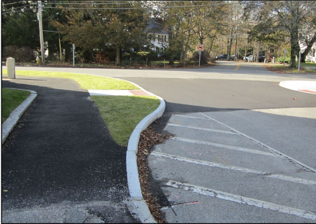
Image 2: Pedestrian bump out with ADA compliant wheelchair ramps at the intersection of Boston Rd. and Lincoln St. in Westford. These improvements to pedestrian safety were part of the Complete Street Town Center Pedestrian Improvements project.
