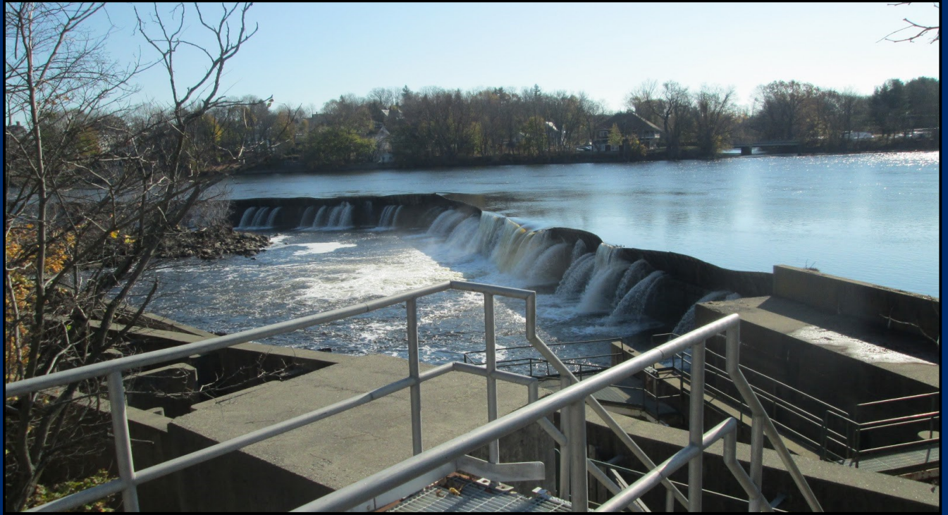
Pawtucket Falls Dam near the O'Donnell Bridge in Lowell MA.
