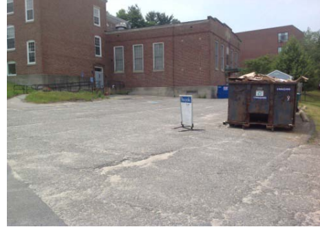
Photo 22: Town Hall Lower Parking Lot (preconstruction)
