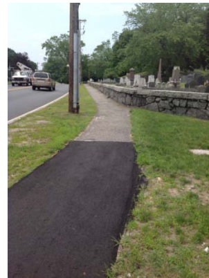
Photo 38: Littleton Rd. Sidewalk
