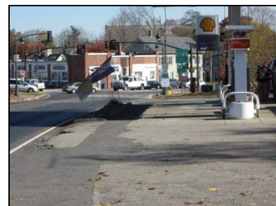
Photo 31: Gap in Sidewalk Network on Littleton Road.
