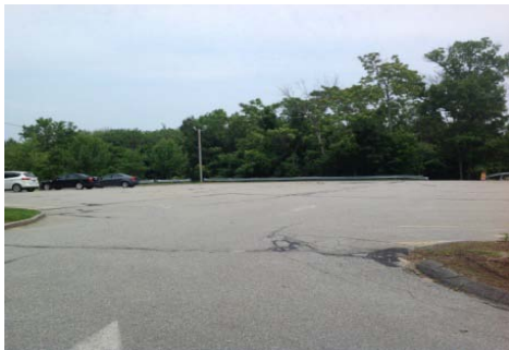
Photo 19: Town Hall Upper Parking Lot (preconstruction)
