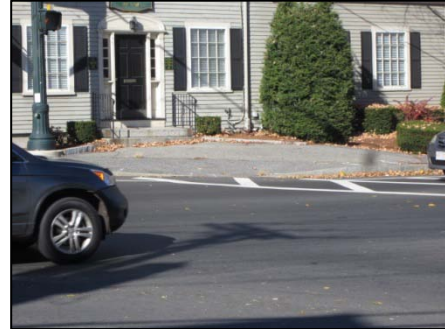
Photo 34: Poor curb cut at NW corner of Chelmsford Street and Billerica Road intersection in Central Square.
