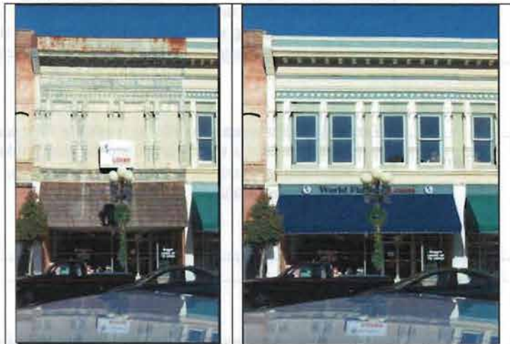
Example restoration of historic commercial building by removing conflicting alternations elements and restoring original architectural elements
