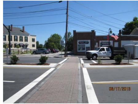
Photo 36: Obstructed pedestrian signal at BFRT crossing
