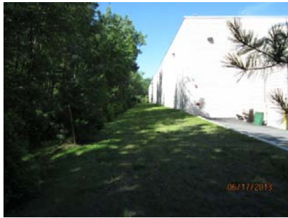
Photo 4: Fire lane behind Stop&Shop
