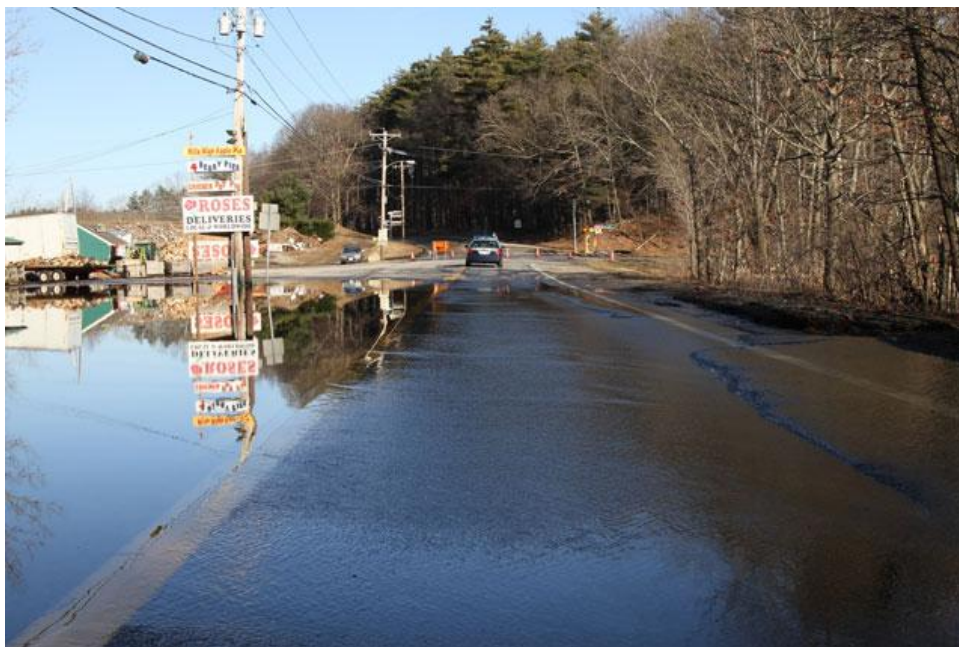
2010 Roadway flooding along Route 119 in Pepperell
