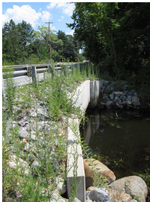
East Street/Strongwater Brook crossing after project completion
