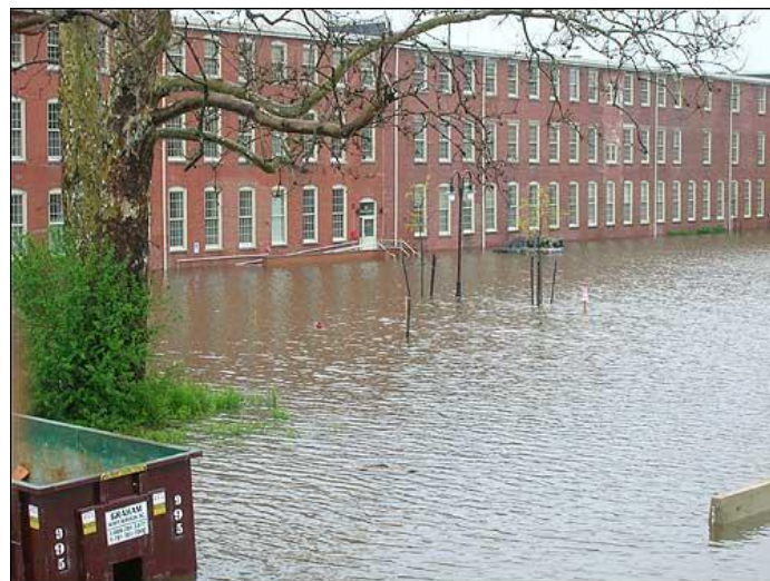
Flooding at the Lawrence Mills in Lowell in 2007
