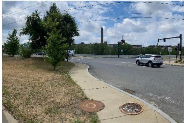
Photo 16: View of Lakeview Avenue at VFW Highway. Source: Road Safety Audit.
