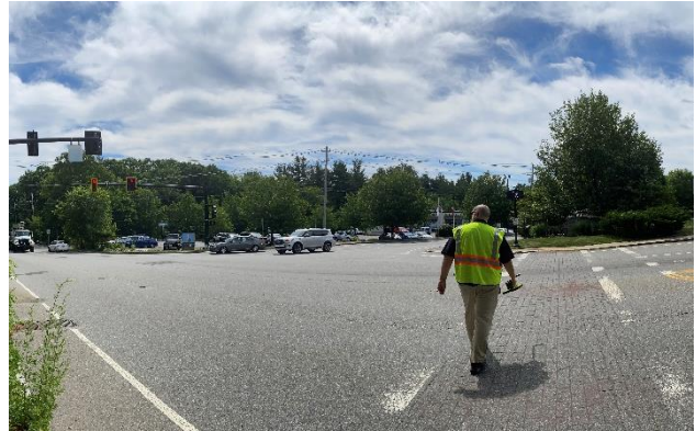
Photo 4. East St/Dascomb Rd at Shawsheen St (looking east after improvements). Source: Site visit.
