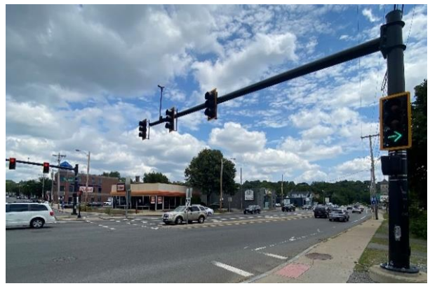
Photo 18: VFW Highway at Bridge Street (looking east after improvements). Source: Road Safety Audit.
