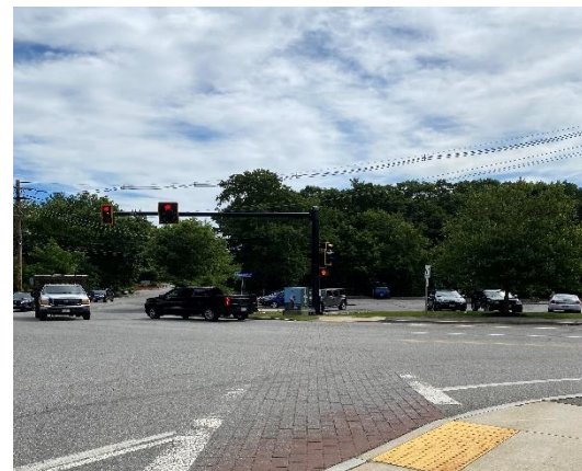
Photo 8. Widened intersection after improvements to prevent potential conflict between turning vehicles and through vehicles. Source: Road Safety Audit.
