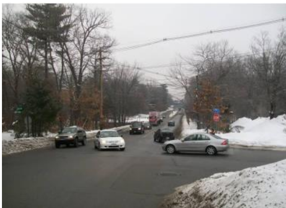
Photo 7. Potential conflict between turning vehicles and through vehicles before improvements. Source: Road Safety Audit.
